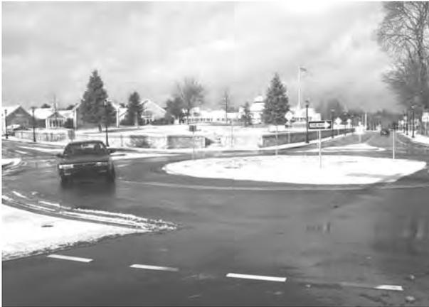
***Roundabouts are intersection control measures that provide speed reduction.***
